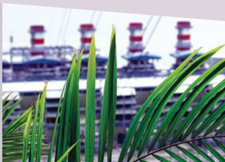
Above: Lumut power plant, Malakoff, Malaysia
