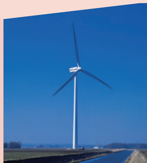
Above: Wind farm, Australia
