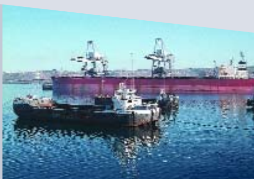
Above: Coal delivery facility, Pego, Portugal
