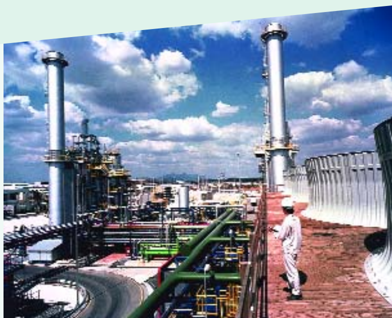
Above: Thai National Power (Pluak Daeng), Thailand
