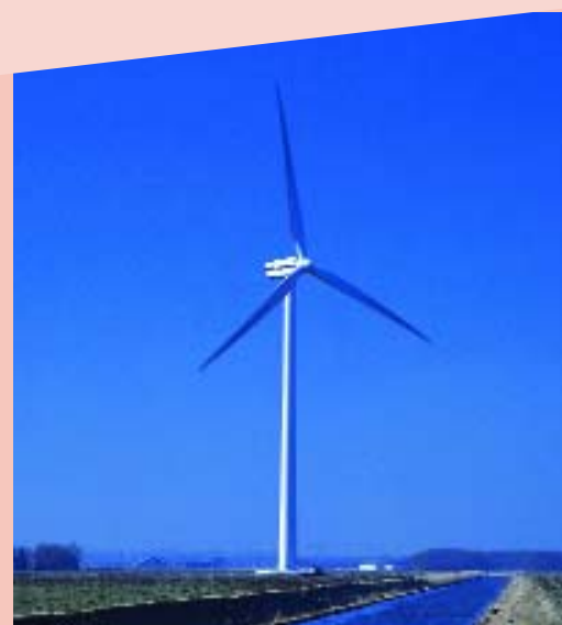
Above: Wind farm, Australia
