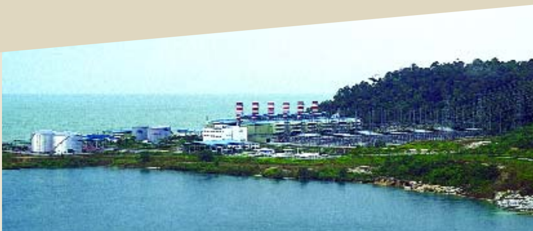
Above: Lumut power plant, Malakoff, Malaysia
