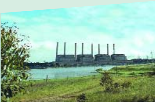
Above: Hazelwood, Australia
